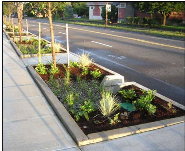
Example BMP: Tree well infiltration pits provide storage, treatment, and infiltration of residential runoff.
